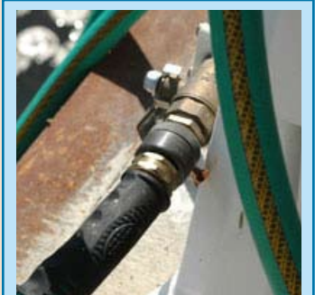
The anti-siphon valve assembly is between the hose spigot and your female hose connector, as shown here.
